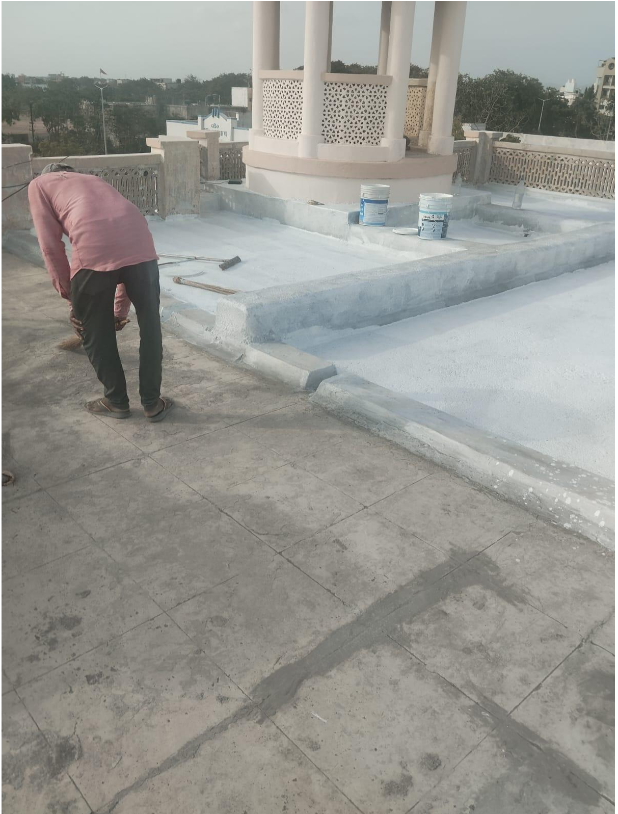
Terrace water proofing
