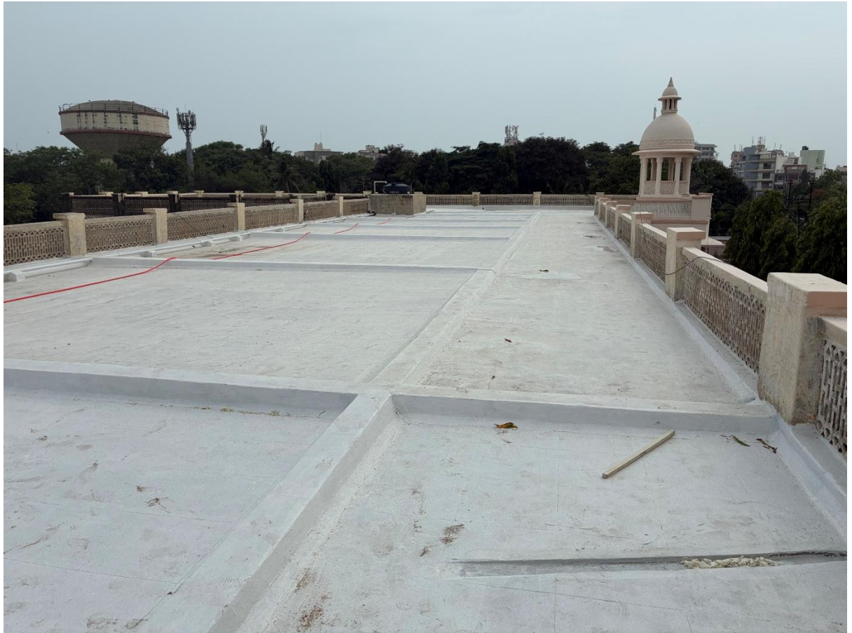
Terrace water proofing
